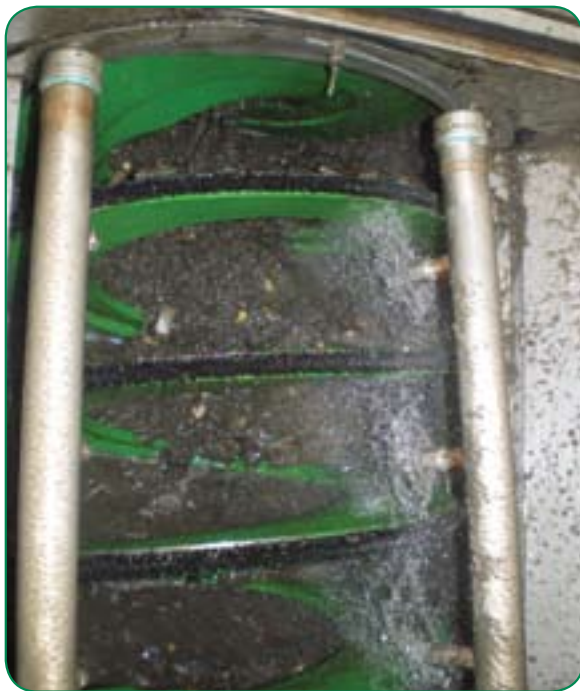
A close-up of the Honey Monster's auger screen and spray wash system. Inorganic solids are captured, cleaned and removed.
