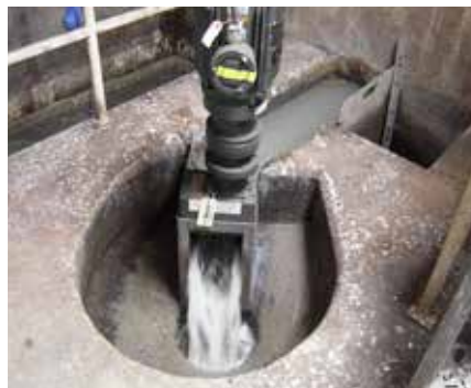
Wet Application 3-HYDRO-C
